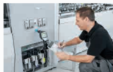
Analysis of compressed air preparation
