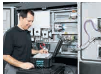
Analysis of compressed air generation
