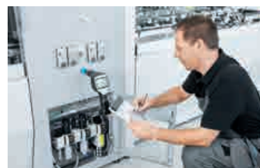
Analysis of compressed air preparation
