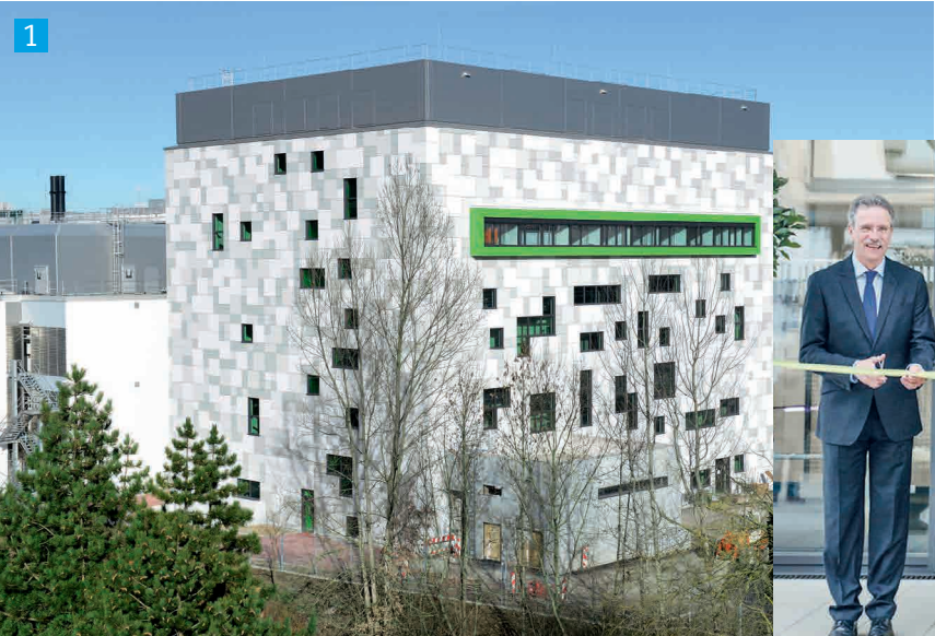
The new K62 Technical Centre at Boehringer Ingelheim in Biberach.
