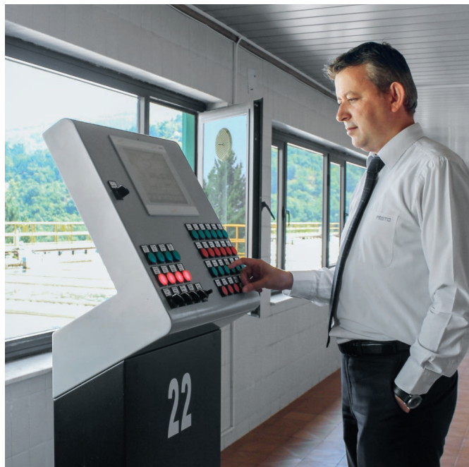
Orhan Ayhan, Festo Process Automation Turkey, checks the new control panel used for standalone (manual or automatic) control of each filter basin
