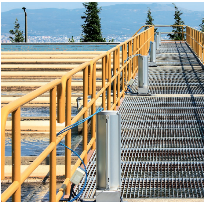
Linear actuators from Festo control the flow into and out of the 28 filter basins
