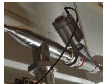
Shut-off control for glycol used in food production
