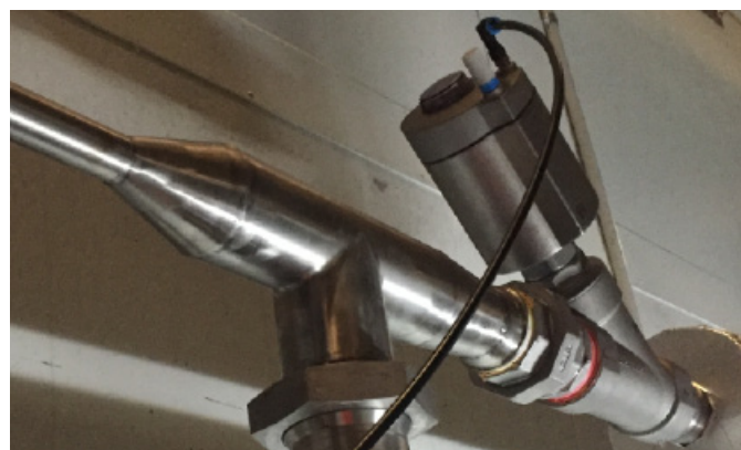
Shut-off control for glycol used in food production
