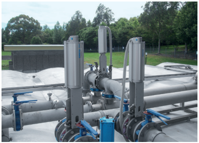
Controlled sluice gate for flowrate of return sludge at a wastewater treatment plant
